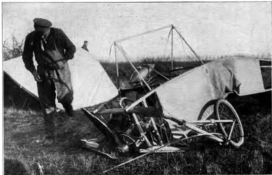
Fig. 46. DeLessep's Machine after Striking an Obstruction
