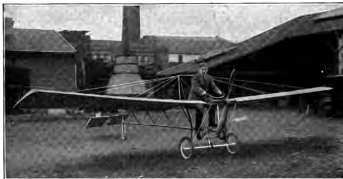
Fig. 38. Aerocycle with Treadle Power for Practice Work
