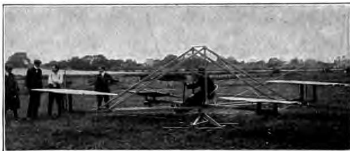
Fig. 37. Monoplane Dummy Used for Practice in Aviation School
