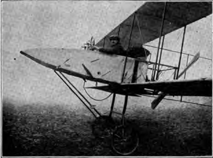
Fig. 39. Voisin Biplane with Double Control for Teaching Beginners
